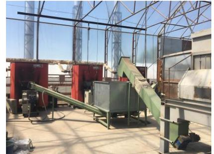
The beneficiary used LEADER funding to install three 300 KW biomass boilers. After extensive search a Hungarian manufacturer was selected and a local entrepreneur was also contracted to construct the building for the boiler room. The investment was completed in March 2014.
